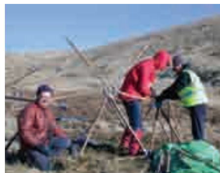
Building a Dome Shelter at 650m for Montane Scrub Planters
