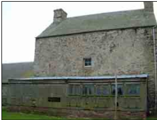
Plate 89 Bastle House and old henhouse at SE boundary of the garden
